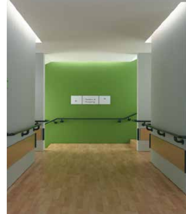
Example of handrails with good visual contrast
