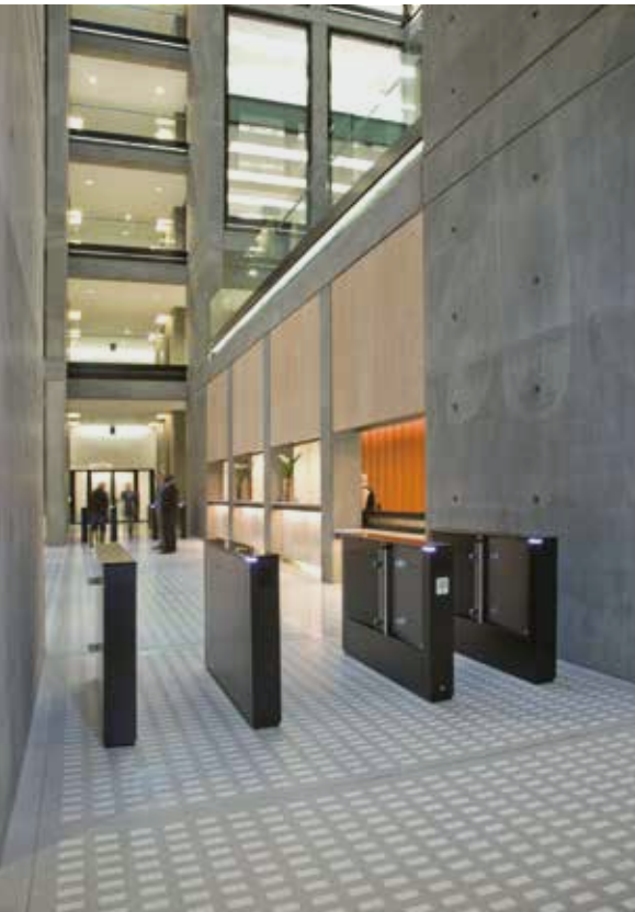
Access control turnstiles
