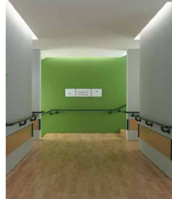
Example of handrails with good visual contrast
